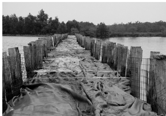
Figure 9-4. Geo-textile crib shortly after installation at the Barataria Preserve. (JELA)
