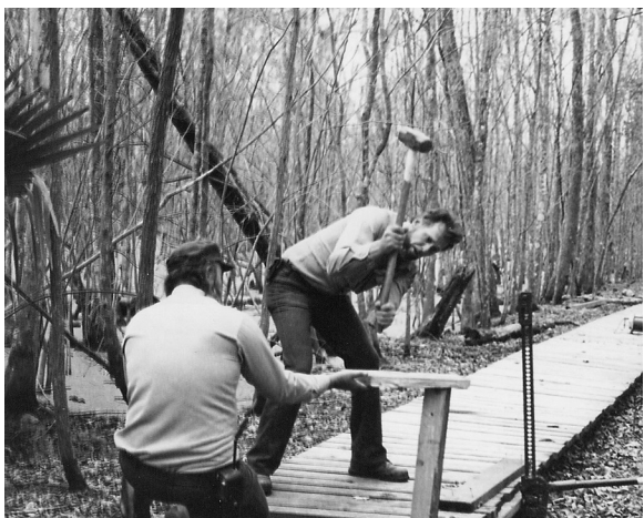
Figure 9-9. Crew building a trail at Barataria, 1980s. (JELA)
