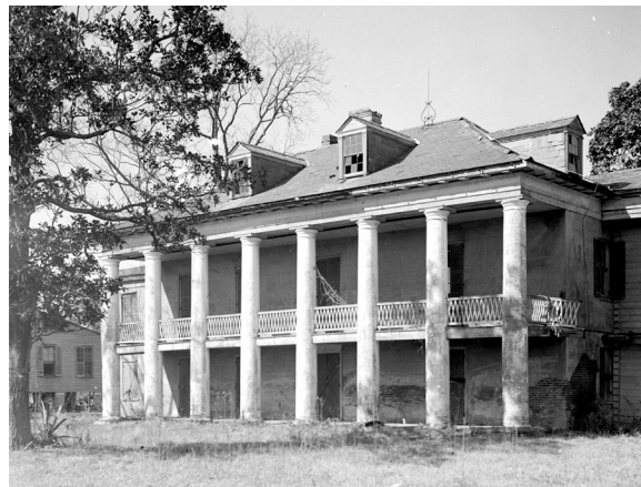
Figure 5-2. Malus-Beauregard House in 1934, before restoration. (HABS)
