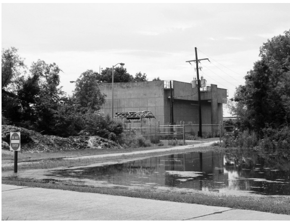
Figure 4-10. Sewage plant on the battlefield, 2008. (author)
