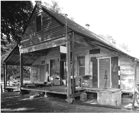
Figure 12-4. Oakland Plantation Store, Cane River. (HABS)
