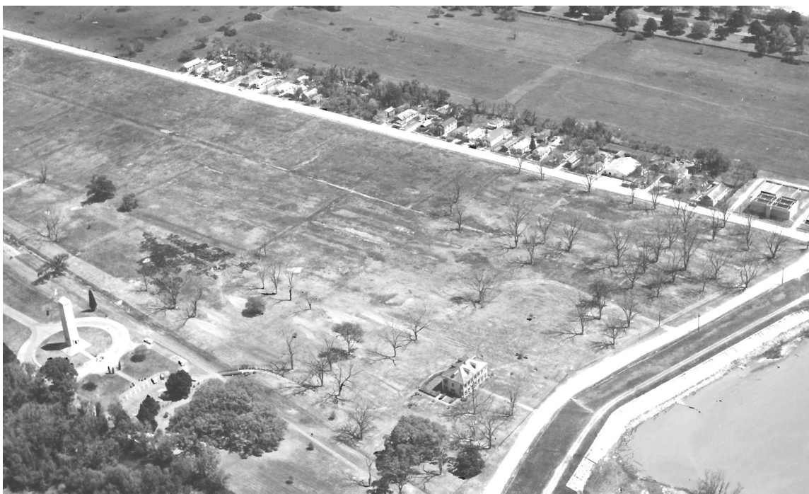
Figure 4-11. Aerial view of monument, Fazendeville, and parish sewage plant. (JELA)
