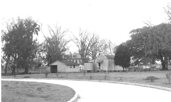
Figure 3-6. Caretaker' house on Chalmette Monument grounds, 1934. (JELA)
