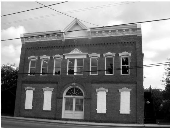
Figure 11-7. Percy Lobdell Building, Thibodaux. (author)
